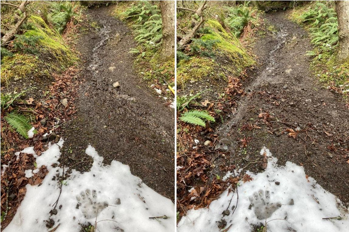
An example of waterbar maintenance on Trail 311. When functioning properly, the waterbar diverts flow from the trail tread to a downslope location. Maintenance is done with hand tools: a McLeod and a round-point shovel.
